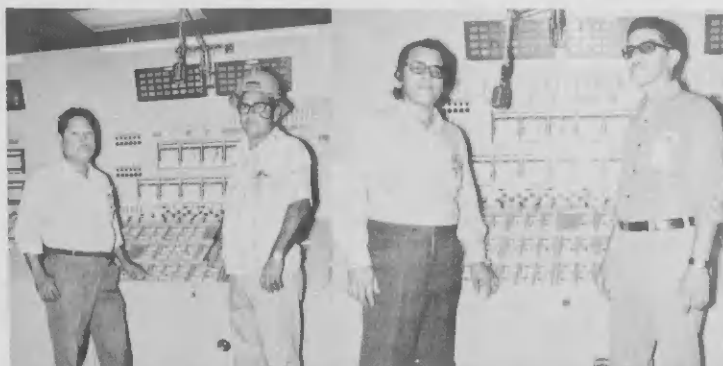
At the control panels for V3AR startup (l to r): J. Wester, T. Tromp, D. Tromp and D. Kelly.
